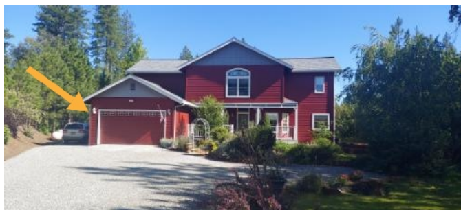
Main Electric Panel Location
